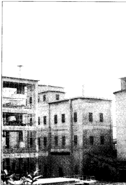
Kien Khe Cement Company - one of enterprises efficiently using capital, land and labour
